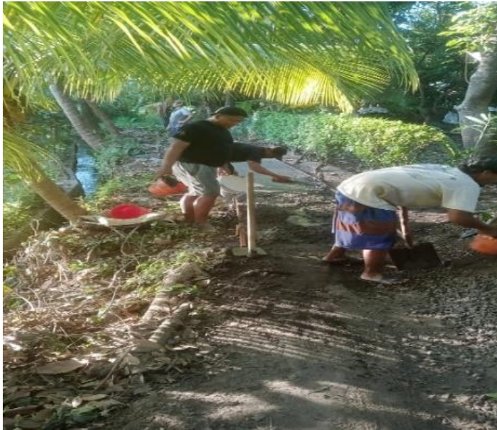
Figure 3. Roadwork with concrete mixture
