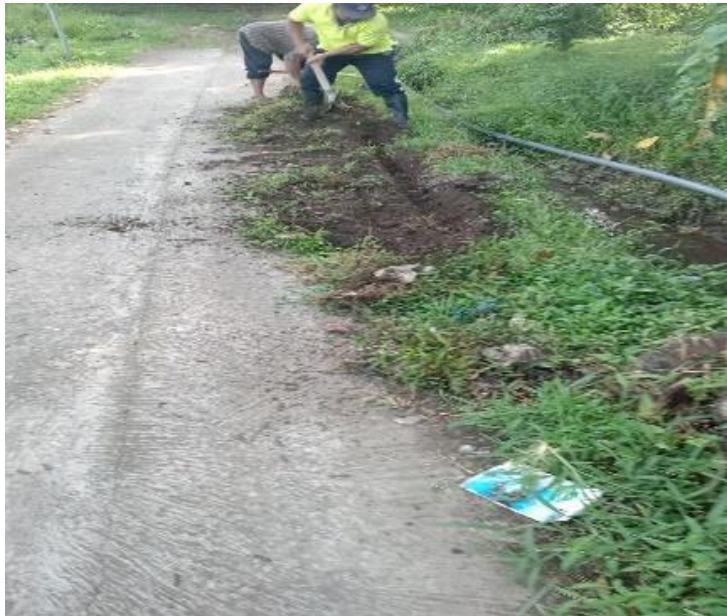
Figure 2. Location of roads repaired with concrete mixture
