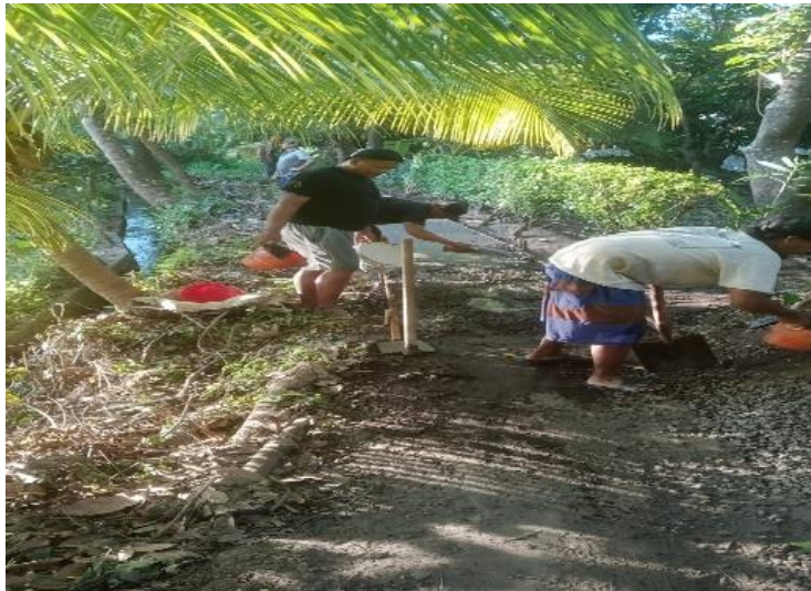
Figure 5. Land leveling work
